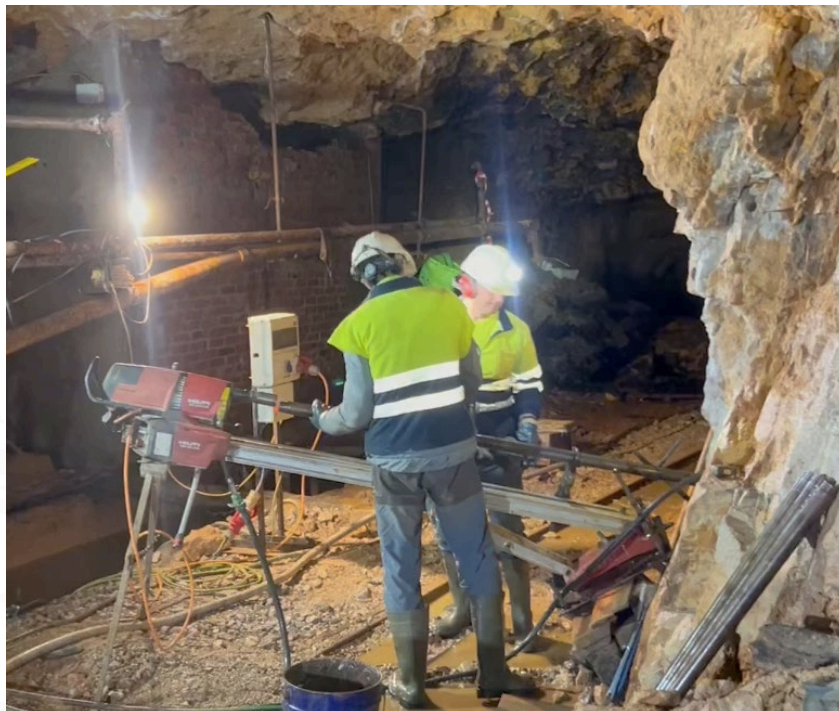
Figure 1. Underground drilling at San Jose Mine gets underway
