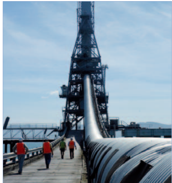
Loading facility at Eden
